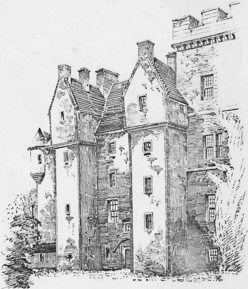
FIG. 915.—Nesbit Castle. View from North-West.
